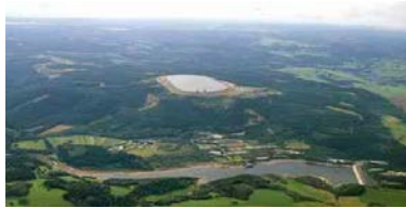
Markersbach: 1050 MW, 4 GWh
