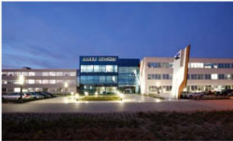
Baker Hughes' Celle Technology Center
